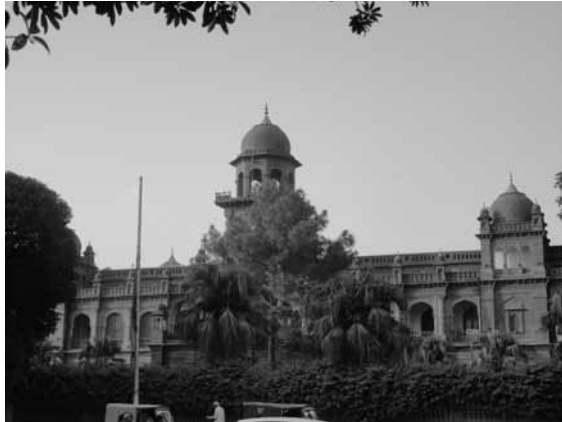
An outside view of Lahore's famous University old campus. Mixing colonial as well as Mughal style buildings.
